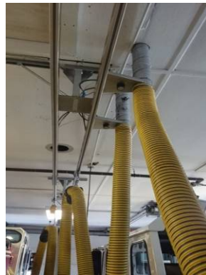
Image 10 – Apparatus Bay PlymoVent System
