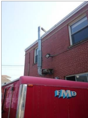
Image 8 – Apparatus Bay Sidewall Exhaust Fan
