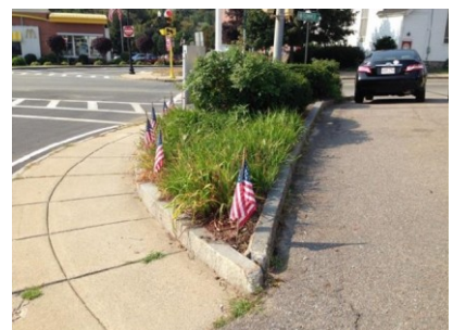
Image 13: Vertical Granite Curbing
