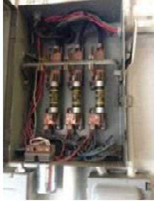
Image 4 – Three Phase Disconnect Switches
