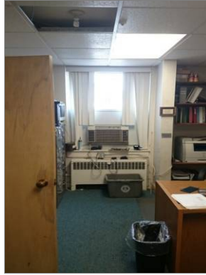
Image 6 – Typical Window AC & Convactor
