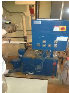
Image 3 – Condensate Receiver
