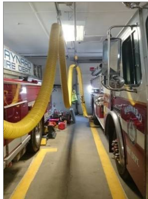
Image 9 – Apparatus Bay PlymoVent System
