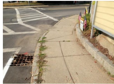
Image 5: Drainage Manhole & Catch Basin in Intersection of Summer St & Acton St
