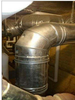
Image 2 – Boiler Vent
