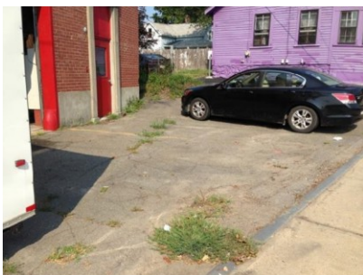
Image 11: Cracks & Vegetation in Parking Lot
