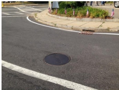
Image 3: Drainage Manhole and Catch Basin in Acton St
