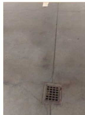
Image 12 – Apparatus Bay Floor Drains
